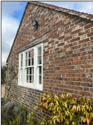
Photograph 3. The south side of the shed.
