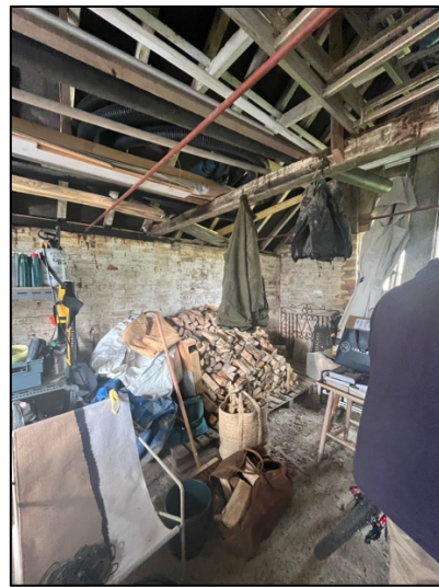
Photograph 15. The opposite side of the shed, interior with wooden crossbeams.
