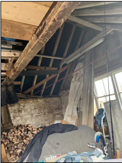
Photograph 20. The roof from the inside of the shed.
