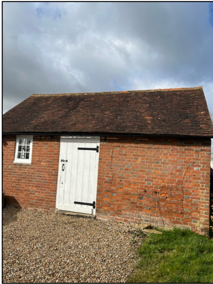
Photograph 1. The front, eastern side of the shed.
