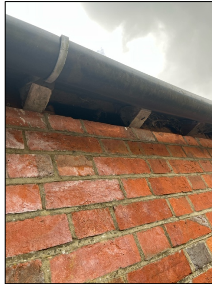
Photograph 13. The soffits and eaves on the west side of the shed.
