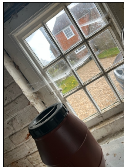
Photograph 17. The window on the western side of the shed, facing the main dwelling. Window providing natural light into the property.
