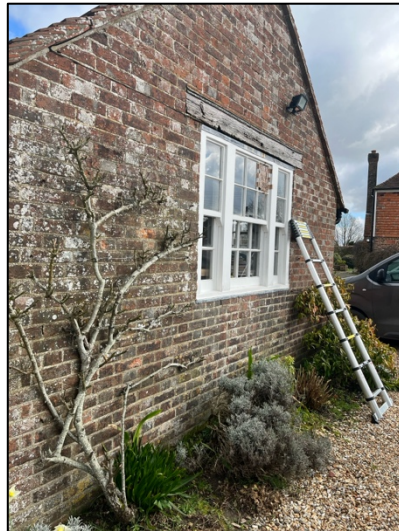
Photograph 4. The southern side of the shed.
