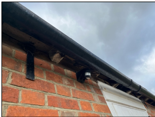
Photograph 8. The soffits and eaves of the shed.
