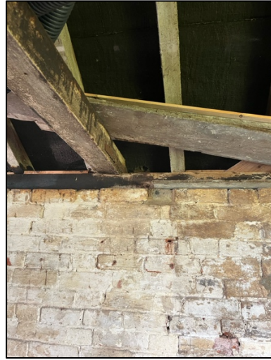
Photograph 19. The roof from within the shed, showing the bitumen lining.
