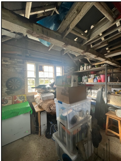
Photograph 14. The inside of the shed, with wooden crossbeams.
