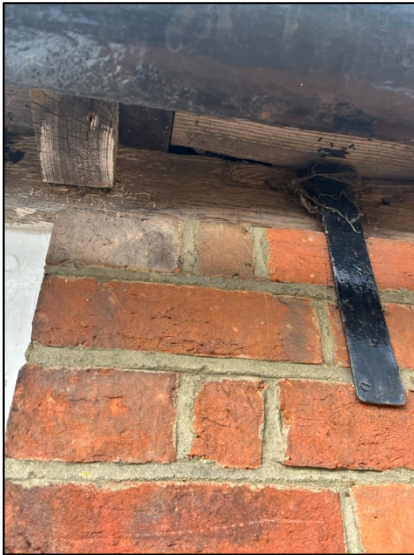
Photograph 12. The eaves and soffits on the west side of the shed.
