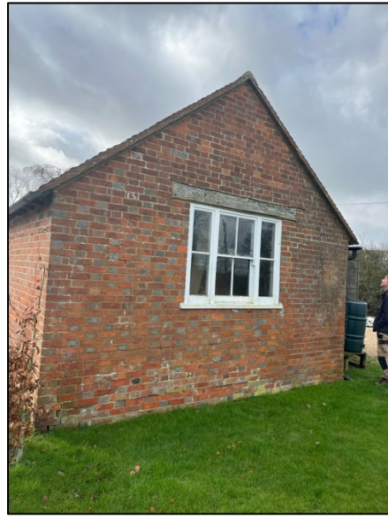
Photograph 2. The rear, northern side of the shed.
