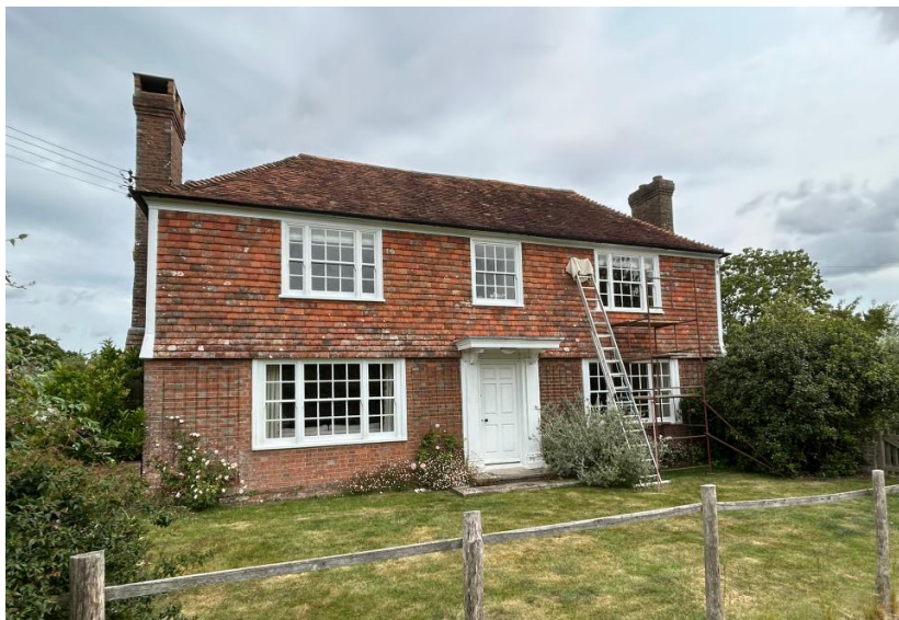
Figure 1. The principal Elevation of Balcony House, this faces South towards Brook Street.
