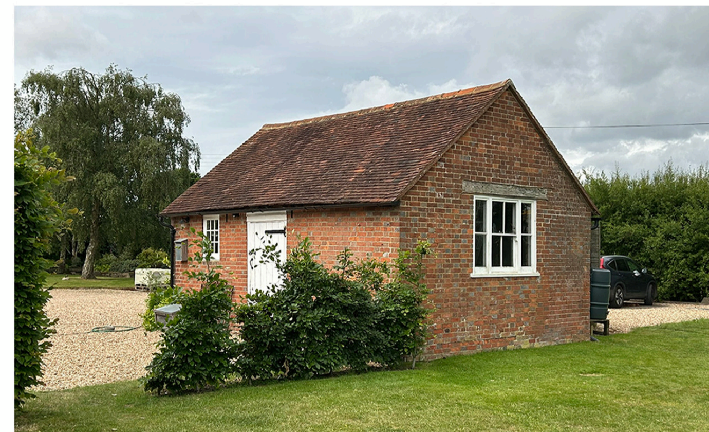
Photo 3 - North-Easterly view of the potting shed
