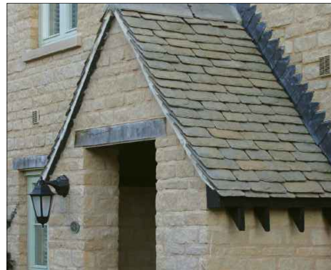
Bradstone or similar stonework with black exposed rafter feet
