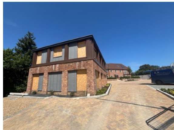
Building A south west elevation
