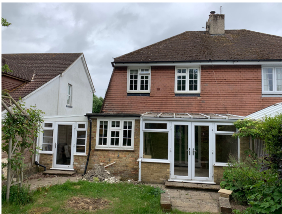
Plate 2 Existing rear elevation viewed from north-east.
