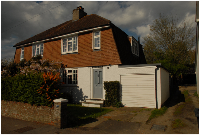
Plate 1 Existing front elevation viewed from south
