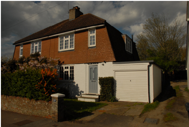
Plate 1 Existing front elevation viewed from south
