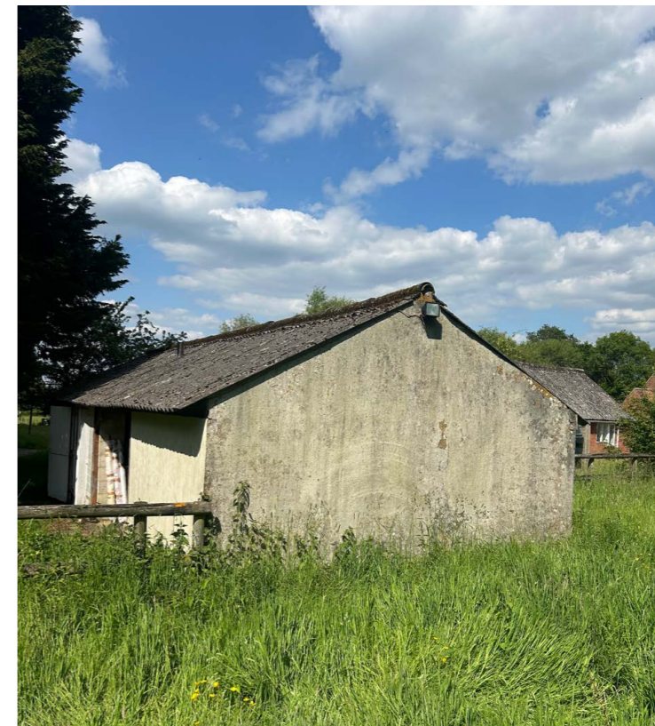
4. View to the rear of the store
