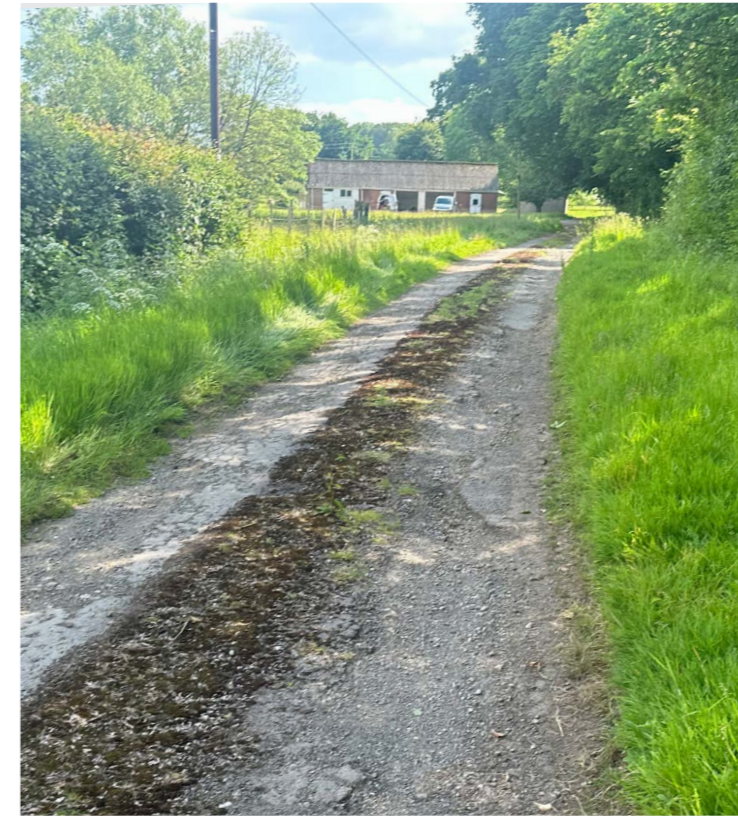
2. View to store from access road
