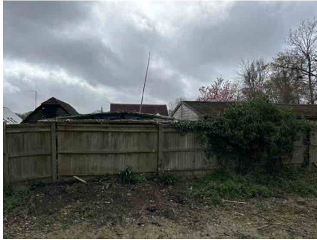
26. Further view of timber fencing on the boundary with site.
