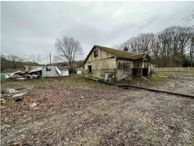
4. View of existing derelict cottage on site.
