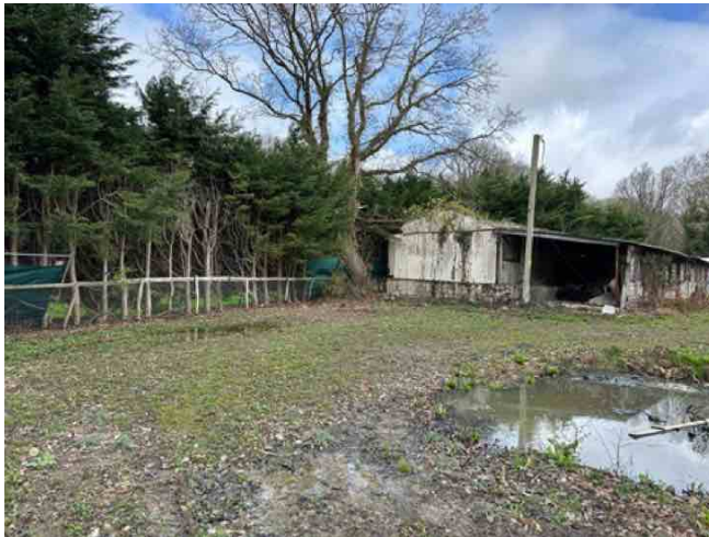
11. Further view of steel frame barn, note trees forming natural barrier.
