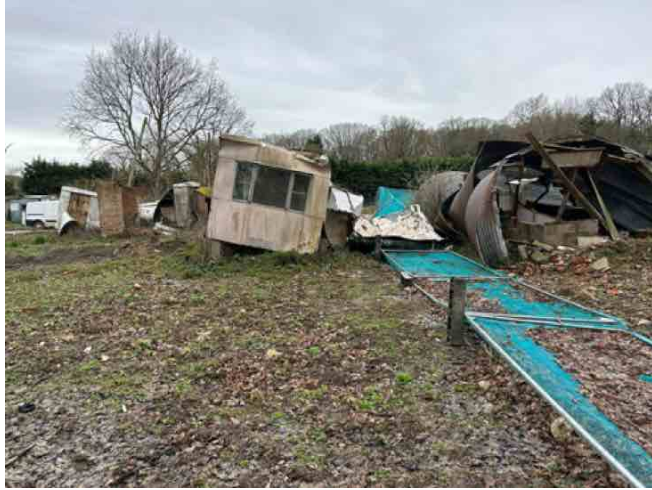
19. Further evidence of the decay with derelict outbuildings, storage units and mobile facilities.
