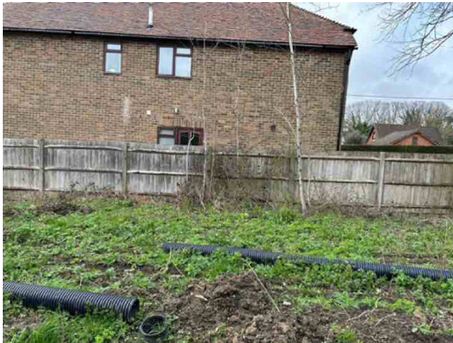
17. Taken from within the lane and looking at Grisbi and existing fencing. Lane to be re-landscaped with SUDs driveway and parking for visitors.
