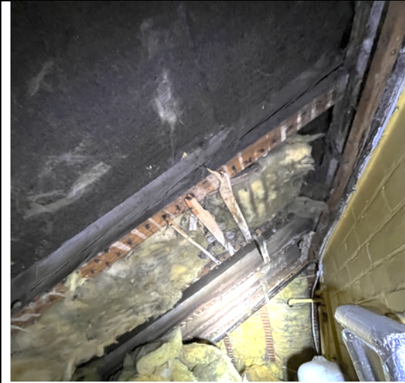
Photo 3. 1F felt lining to roof and partial rock-wall insulation to roof void above east aspect lean-to section
