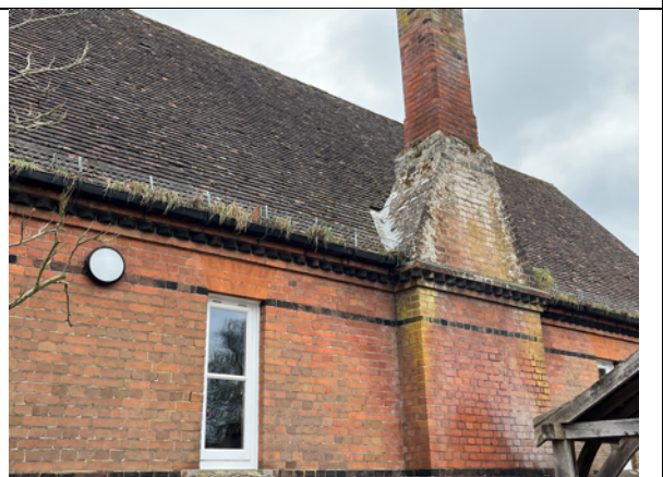
Photo 8. North elevation of main building, with a few gaps under tiles, but no gaps in brickwork, no soffits, and no access to internal void at eaves level
