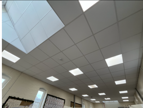
Photo 4. False ceiling to northern section of building, with no access into roof void above
