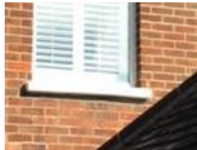
Stone Cills painted white (to match existing at 3 Brickfield Cottages)
