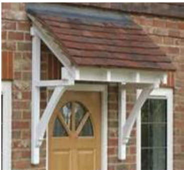
Timber canopy with tiled roof
