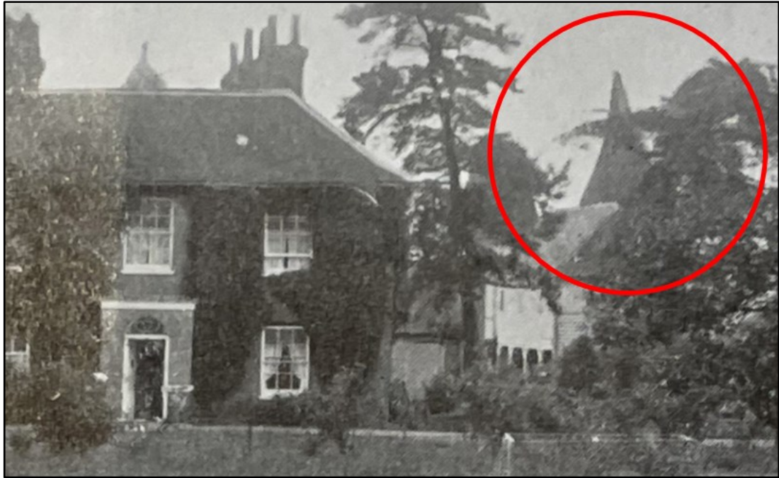
FIGURE 7: PHOTOGRAPH TAKEN FROM THE FRONT GARDEN OF DUESDEN SHOWING DUESDEN OAST
