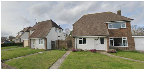
Figure 1: Nos.10, 8 and 6 Homewood Road (l-r)
