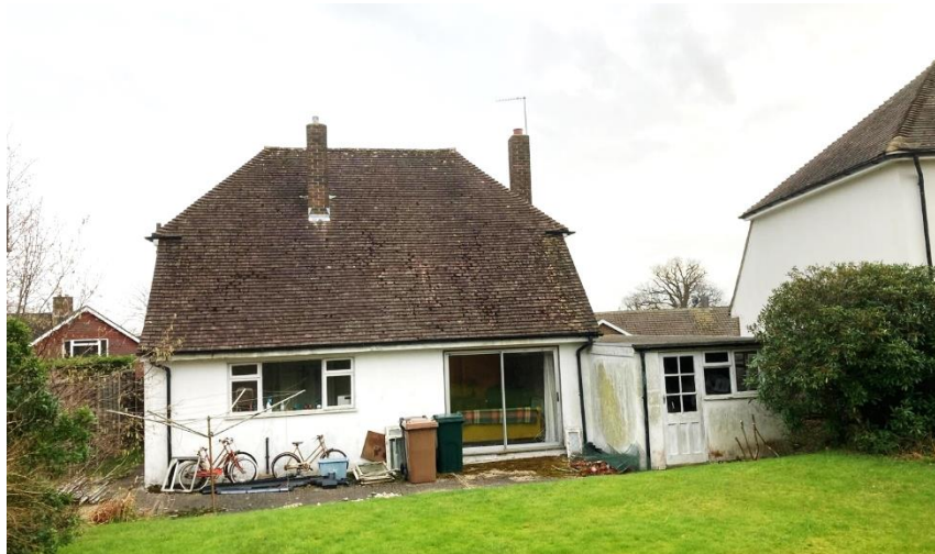
Figure 6: No.8 Homewood Road rear
