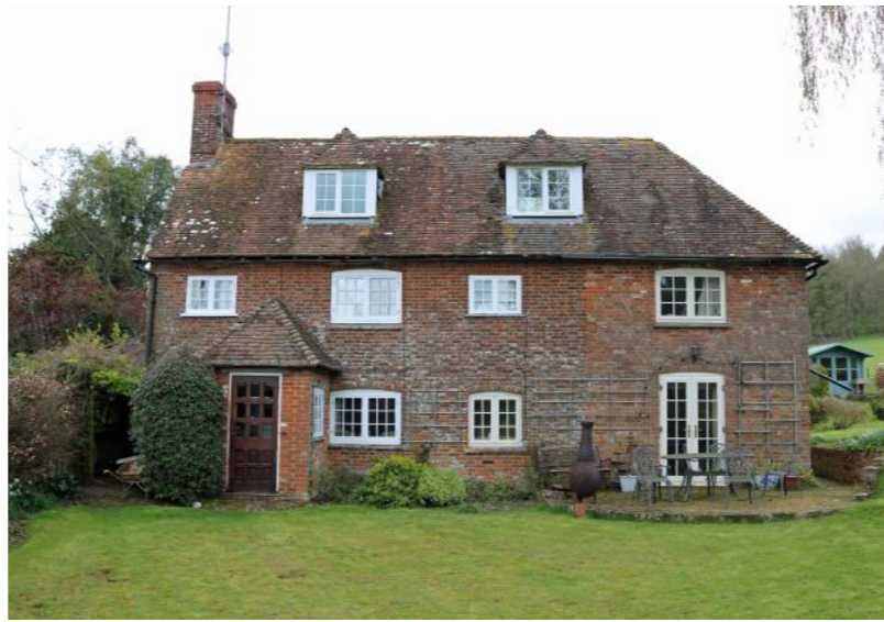
B HUNTSTREET COTTAGE FROM SOUTH
