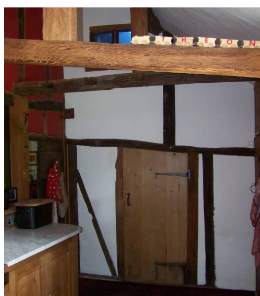
Figure 21: Former Extension Wall
