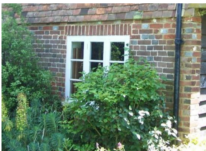
Figure 14: Dragon Post Figure 15: Glazed-Headed Flemish Bond
