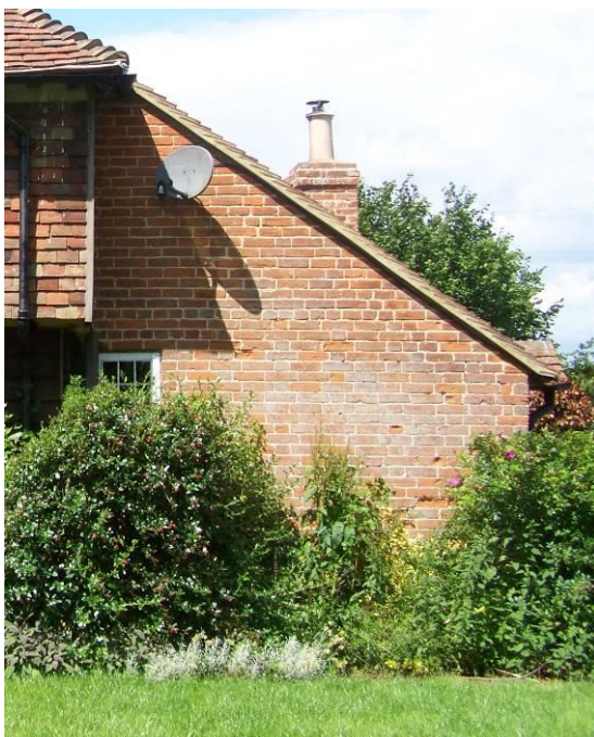
Figure 16: Flemish Bond (to jetty level) Figure 17: English Bond, Segmental Arch
