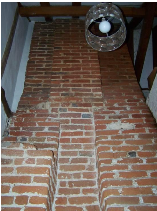
Figure 22: Chimney Stack, Stairwell
