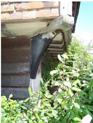
Figure 14: Dragon Post Figure 15: Glazed-Headed Flemish Bond
