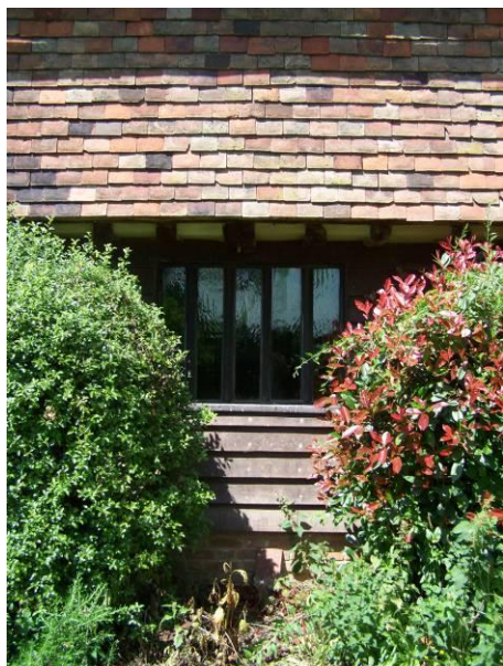
Figure 18: Timber Mullioned Window
