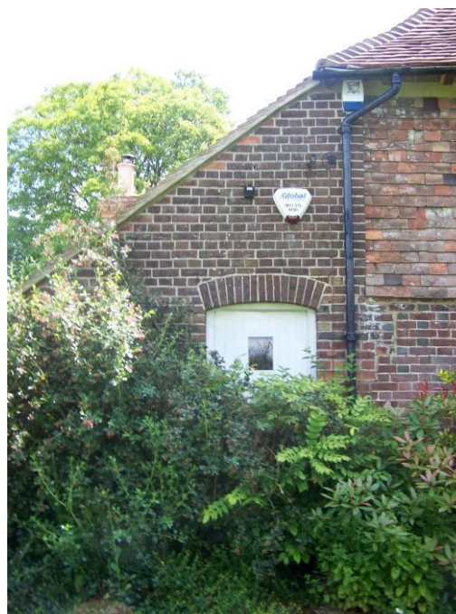
Figure 16: Flemish Bond (to jetty level) Figure 17: English Bond, Segmental Arch
