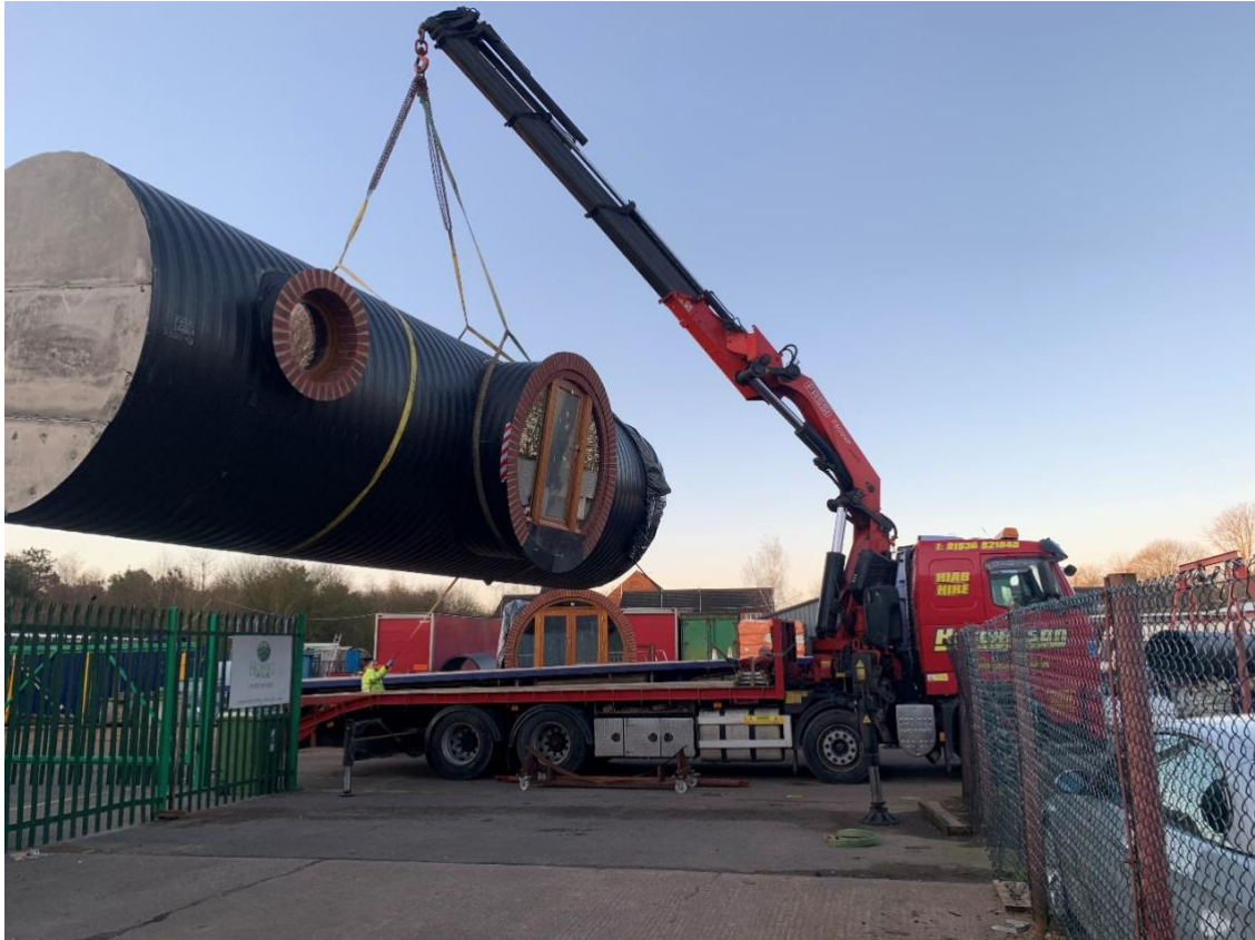
A completed unit arrives on flatbed HGV and is lifted into position by specialist contractor
